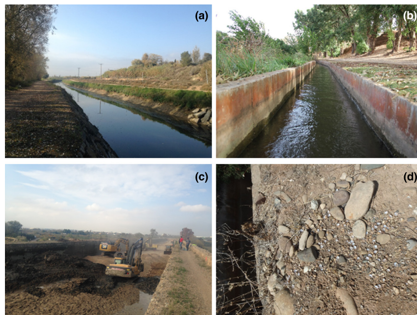
BOX FIGURE B1 Canal Imperial in Aragon (Spain) (a), Bouhlou Irrigation Canal (Morocco) (b), maintenance works in the Canal Imperial (c) and sediment and empty shells of several bivalve species after cleaning activities by farmers in the Bouhlou Irrigation Canal (d)
